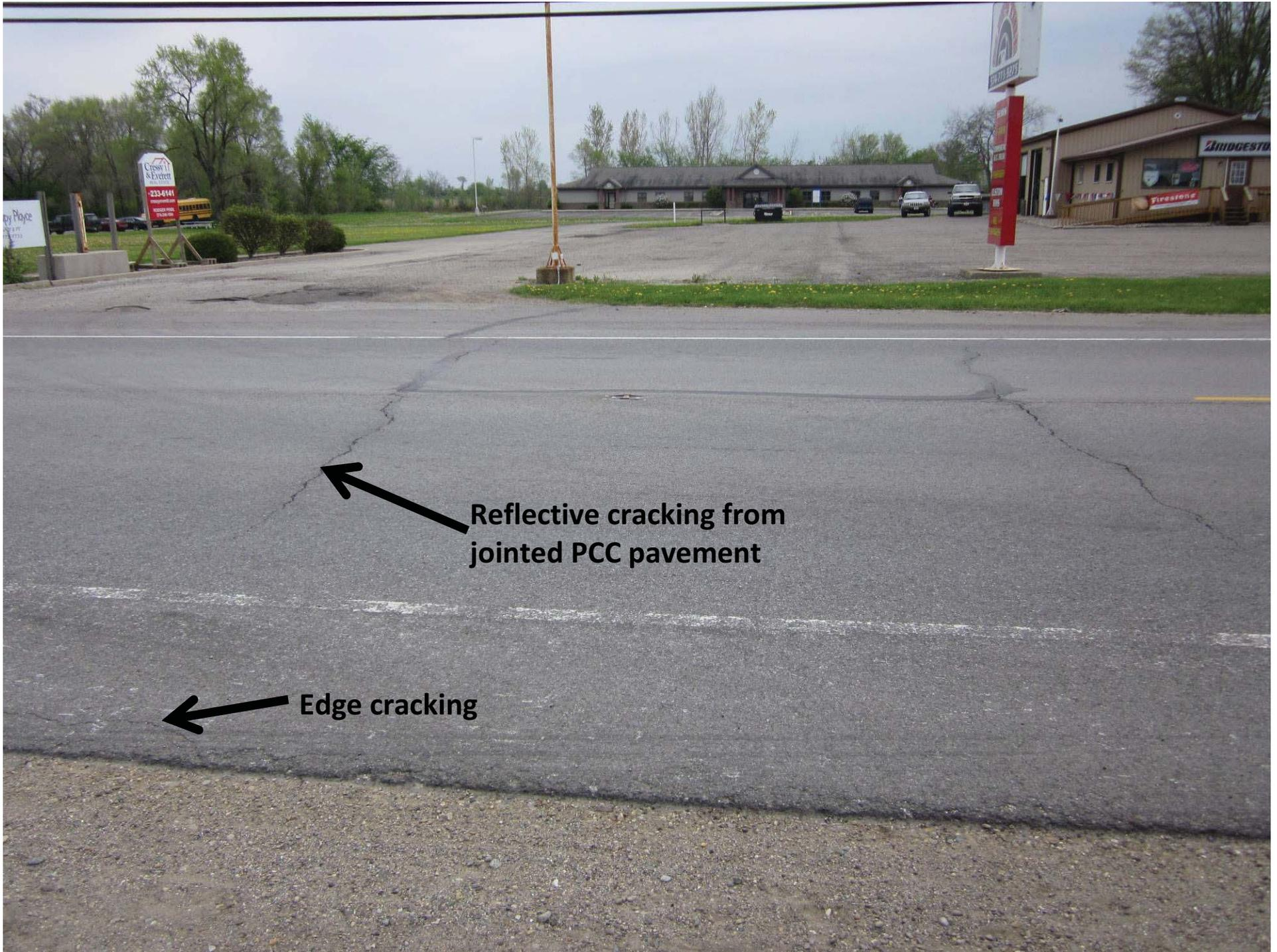
Reflective cracking from jointed PCC pavement
